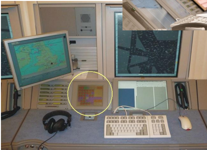
Area Control workstation: ground-ground communications panel highlighted
